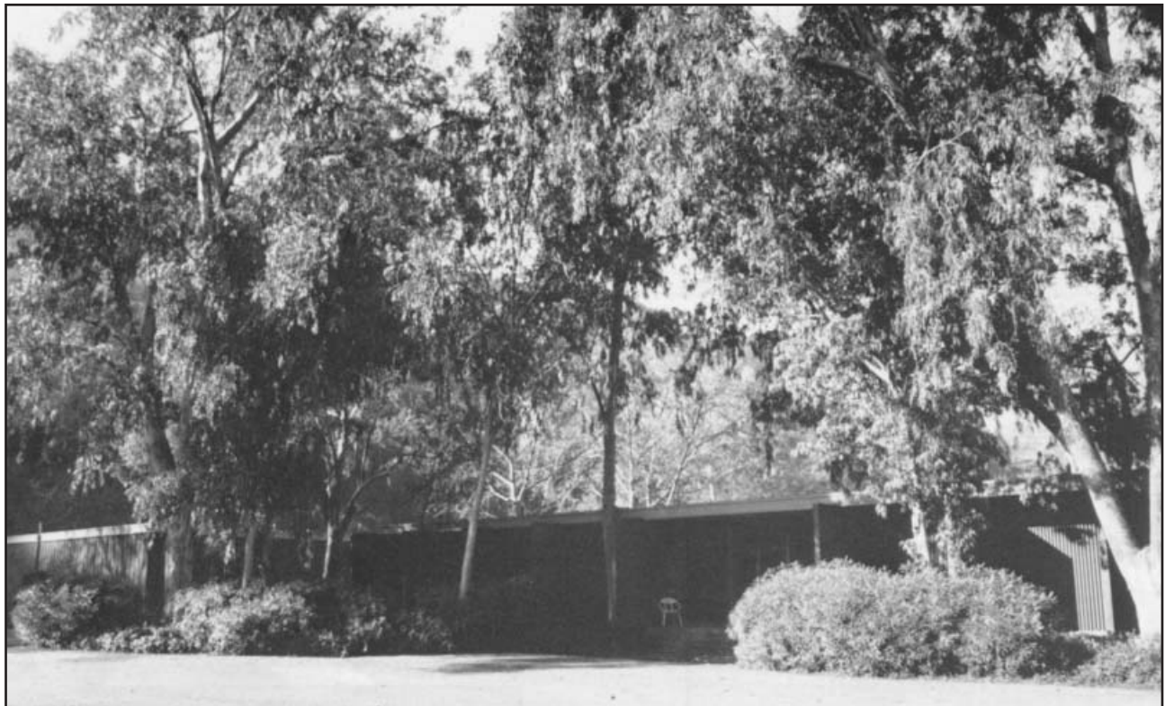
Telonic Berkeley, Inc. manufacturing facility in Laguna Beach, California.
